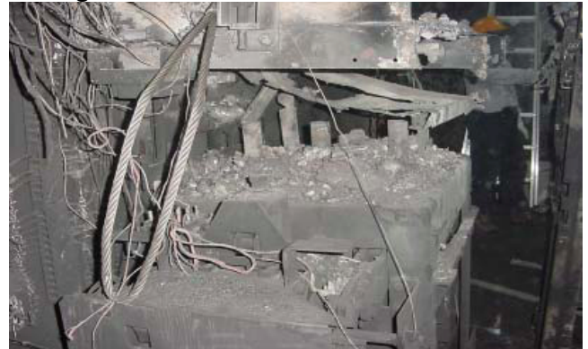
Damaged Breaker
