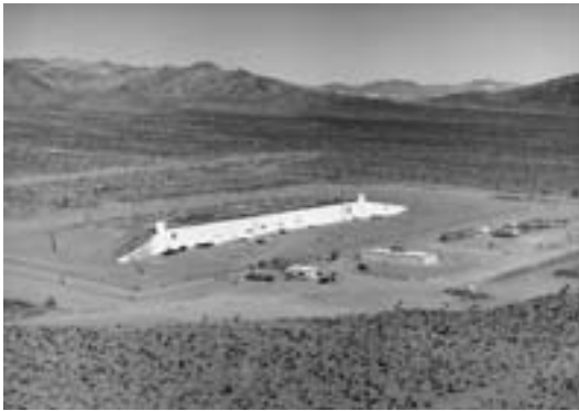
Figure 4.2. The Device Assembly Facility on the Nevada Test Site. A 10,000 m 2 facility, the DAF is designed for security. It is mostly underground, behind the one visible wall with its two guard towers. It was built in the early 1990s for assembly of nuclear explosives before nuclear tests. Recently, DOE moved to the DAF a portion of the 2.8 tons of fissile materials removed from Los Alamos Technical Area 18. 171
