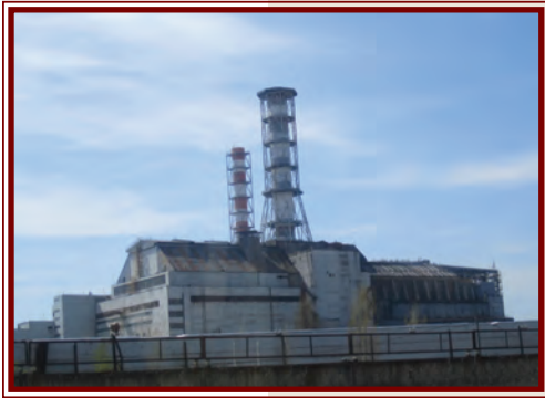
Photo of reactor #4 of the Chernobyl Nuclear Power Plant taken on April 25, 2012. (Source: USC)
