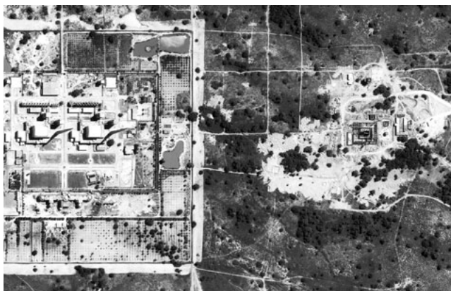
Figure 5. New construction at Pakistan's Khushab site. Khushab-II and -III are visible on the left. Khushab-II began operating in late 2009 or early 2010, and Khushab-III is still under construction. Construction of the Khushab-IV plutonium production reactor is visible on the right. Khushab-I (not shown in the image) has been operating since 1998. Source: GeoEye satellite imagery, 20 April 2011.
