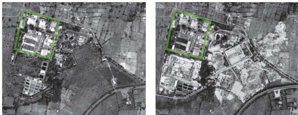
Figure 2. New construction at India's enrichment complex, the Ratehalli Rare Materials Plant, near Mysore in April 2005 (left) and February 2011 (right). The existing enrichment halls are in the upper left
