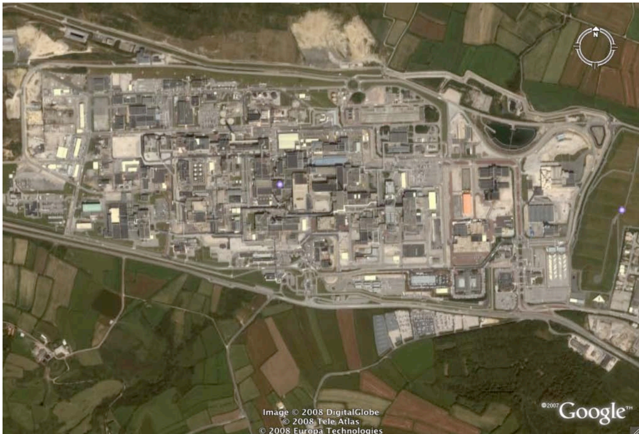
Figure 5. The reprocessing complex at La Hague. The site comprises the old UP2-400 plant and the operating plants UP2-800 and UP3 and their annex facilities (spent fuel storage, waste treatment).
